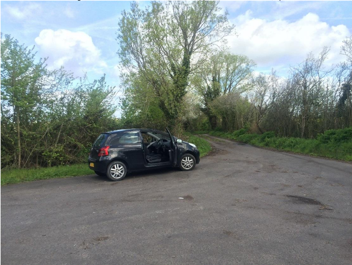
Photo 14: Tarmac turning circle at the north side of the A303, approximate Ch. 2000m, option E4.
