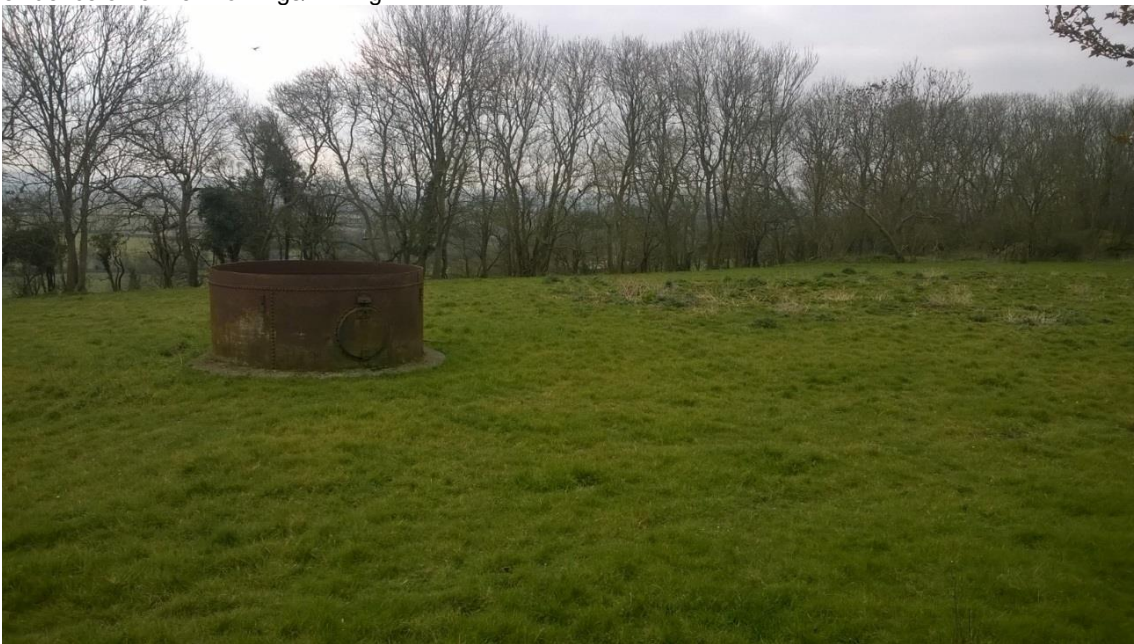
Photo 6: Large steel tank concreted into the ground. The surrounding ground is uneven and hummocky – possible evidence of former workings/infilling.
